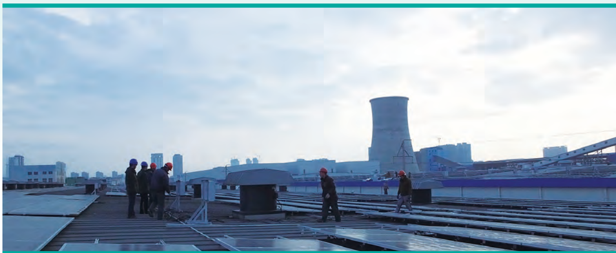
Rongcheng distributed solar station under construction
