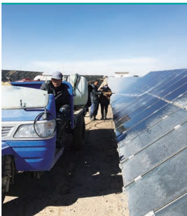
Module clean in progress at Qinghai solar farm
