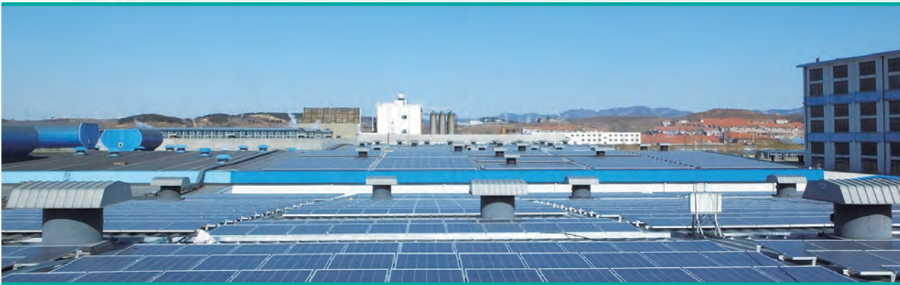
A section of Rongcheng distributed solar station
